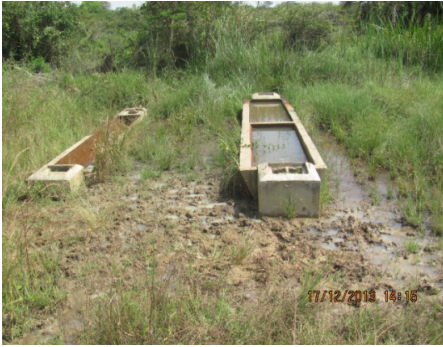
Some of the drinking troughs covered in bushes and with surrounding area water logged.
