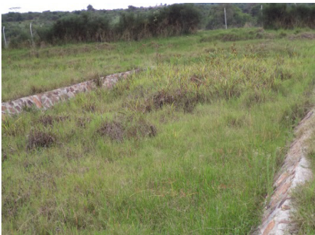
A section of the by-pass channel over grown bush at Obwegyerero valley tank.
