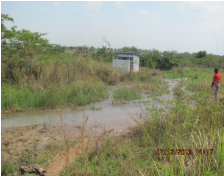
Access route to the toilet at Akwera all submerged in water making the facility unaccessible.
